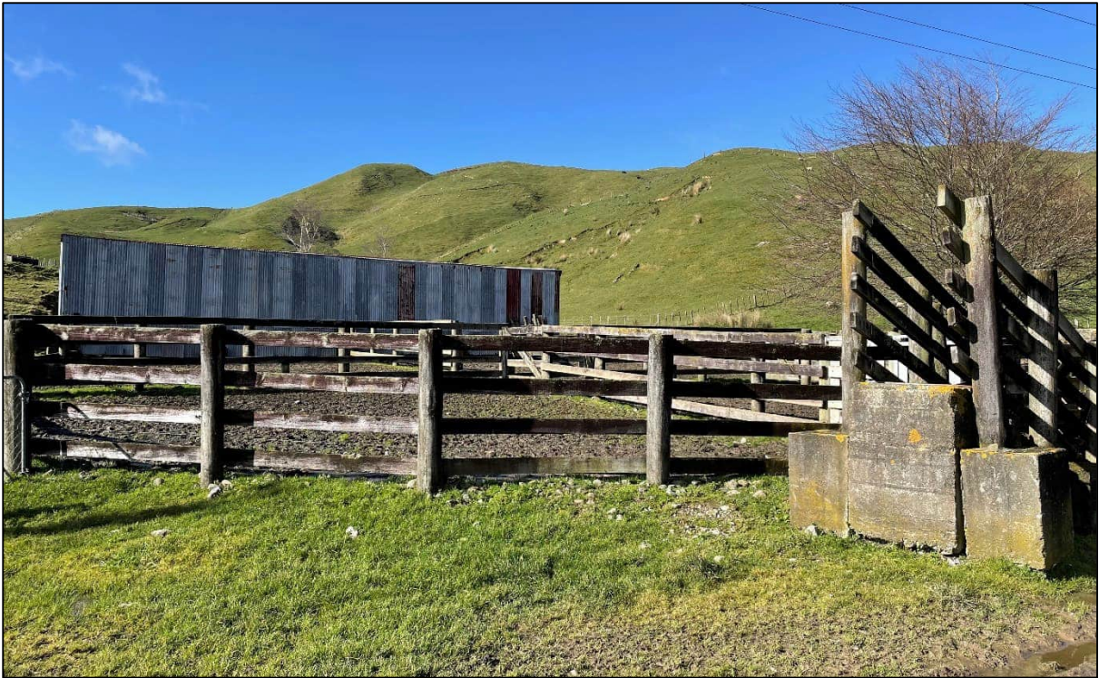
Photograph Appendix B.7: Stockyard and loading ramp adjacent to Old Coach Road. Rear of ancillary shed beyond.
