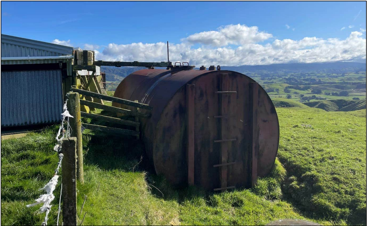
Photograph Appendix B.11: Storage tank used as a water tank, with pipe connected from the roof of the super bin to the tank.
