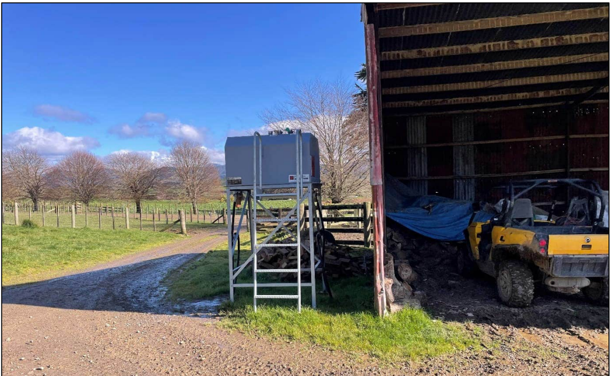
Photograph Appendix B.8: Aboveground storage tank adjacent to south wall of shed. Split tank containing both petrol and diesel.
