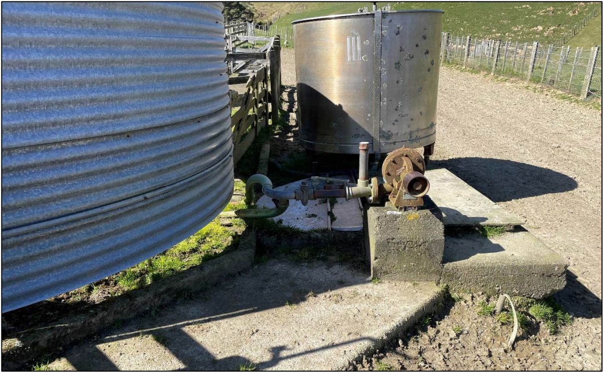
Photograph Appendix B.15: Southern side of sheep dip showing collection sum (with pump) and small mixing tank. The concrete curb bund that surrounds the tank can be seen to the left of the image.
